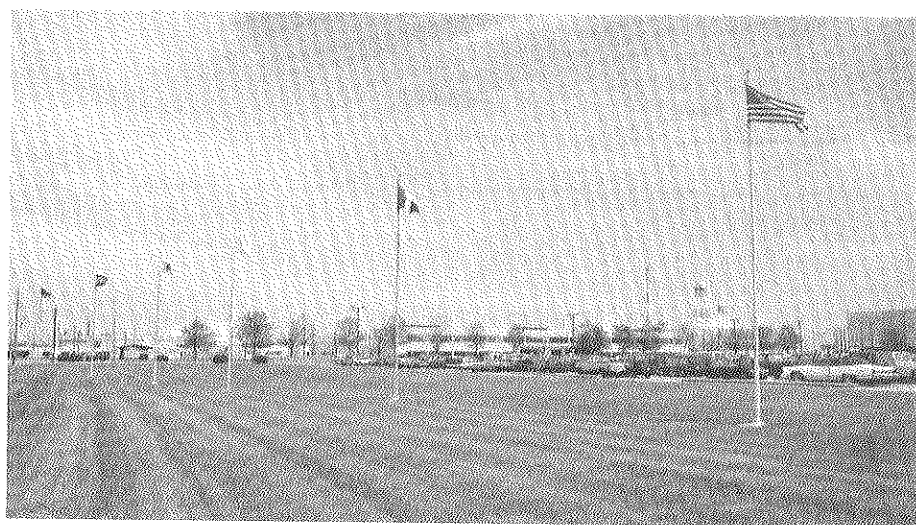
Paducah Gaseous Diffusion Plant Paducah, Kentucky
